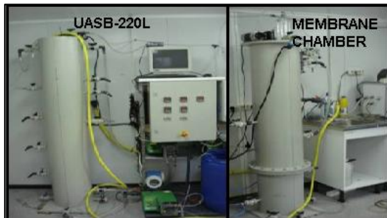
Figure 3. Urban wastewater An-MBR pilot plant. (Valladolid)
