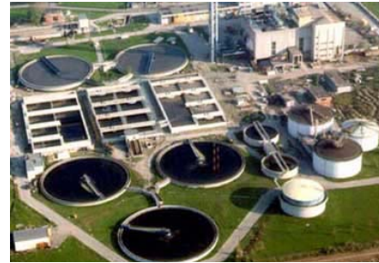
Figure 1. Aerial view of a WWTP
